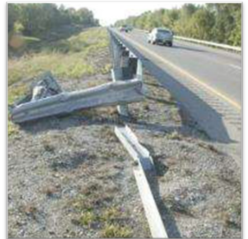
Damaged Guardrail
