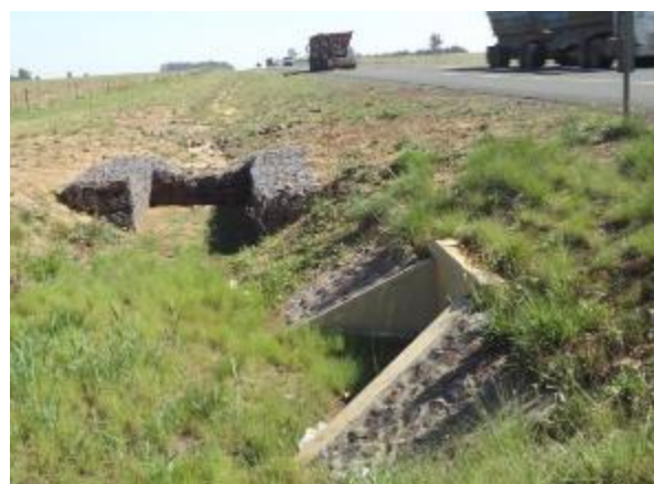
Inlet structures within clear zone
