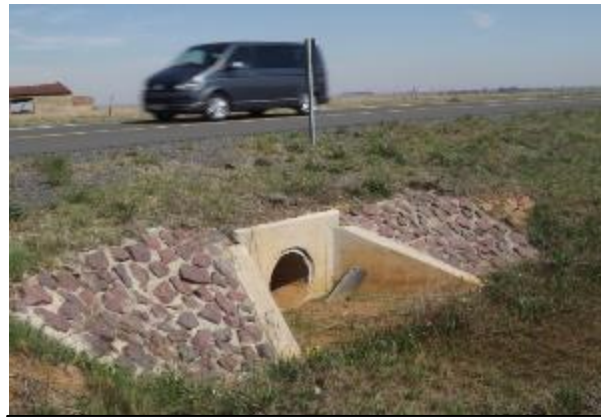
Drainage structure close to road
