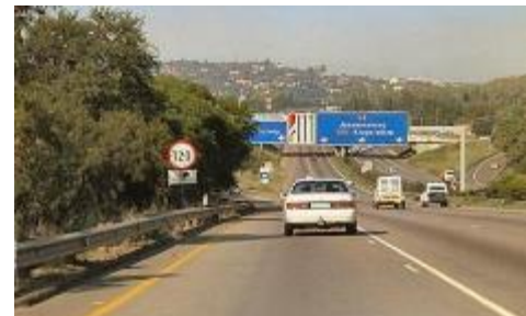
Road sign behind barrier
