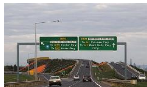
Example of protected gangtry
