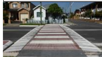
Raised Pedestrian Crossing
