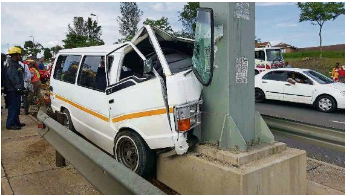
Figure 30: Illustration of Gantry Base in Median
