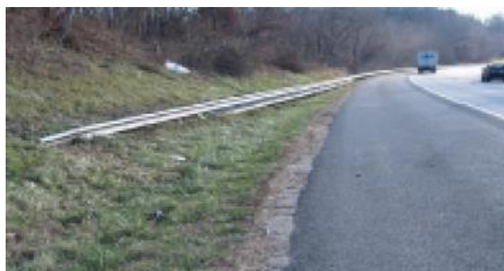
Figure 20: Buried in Backslope Barrier Terminal
