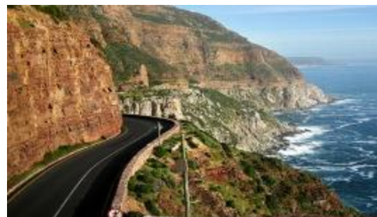
Stone Masonry barrier on Chapmans Peak Drive
