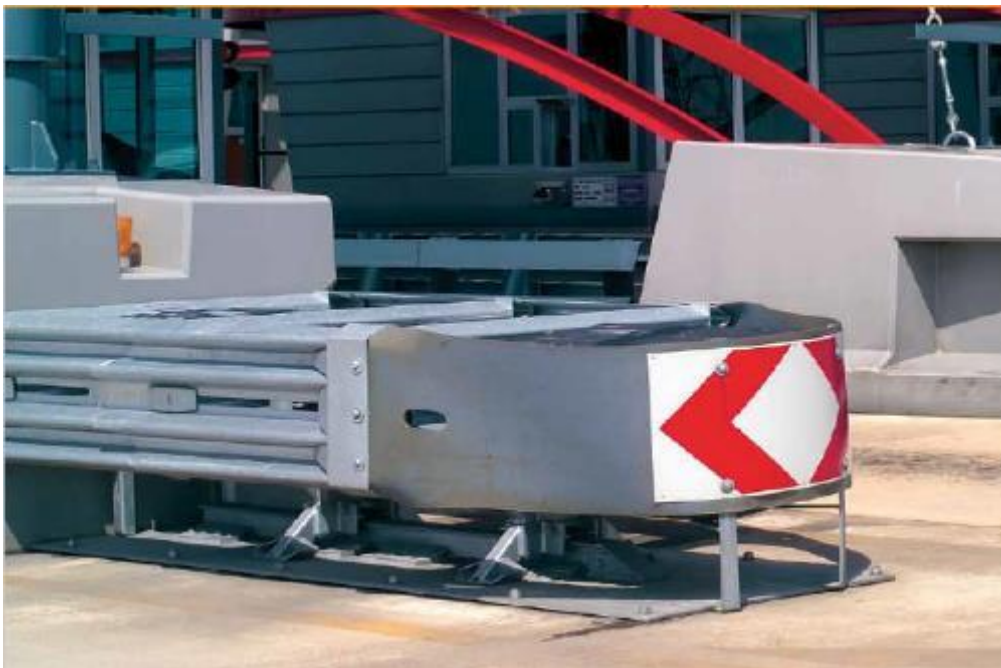
Figure 23: Crash Cushion at Toll Booth
